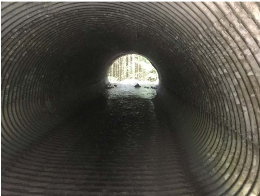
Looking through culvert
